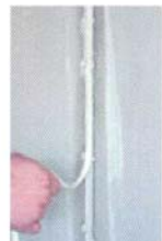
Apply 1/2" tape into the tapered edge
