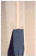
Imbed tape into the tapered edge with the knife's corner
