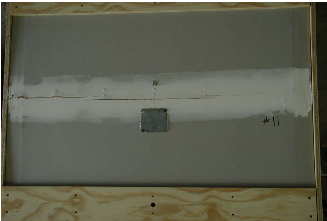
Figure 10 – Tension Failure – ButtTaper joint w/backer failure load = 3028
