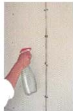
Spray water into space or imbed with diluted spackling compound
