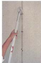
Gradually apply pressure on the space with the ButtTaper
