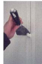
Imbed spackle into the tapered edge with the knife's corner
